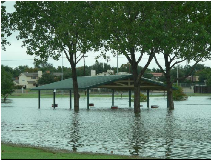
Picture of flooding at Charles Guy Park in Lubbock on September 12, 2008.
